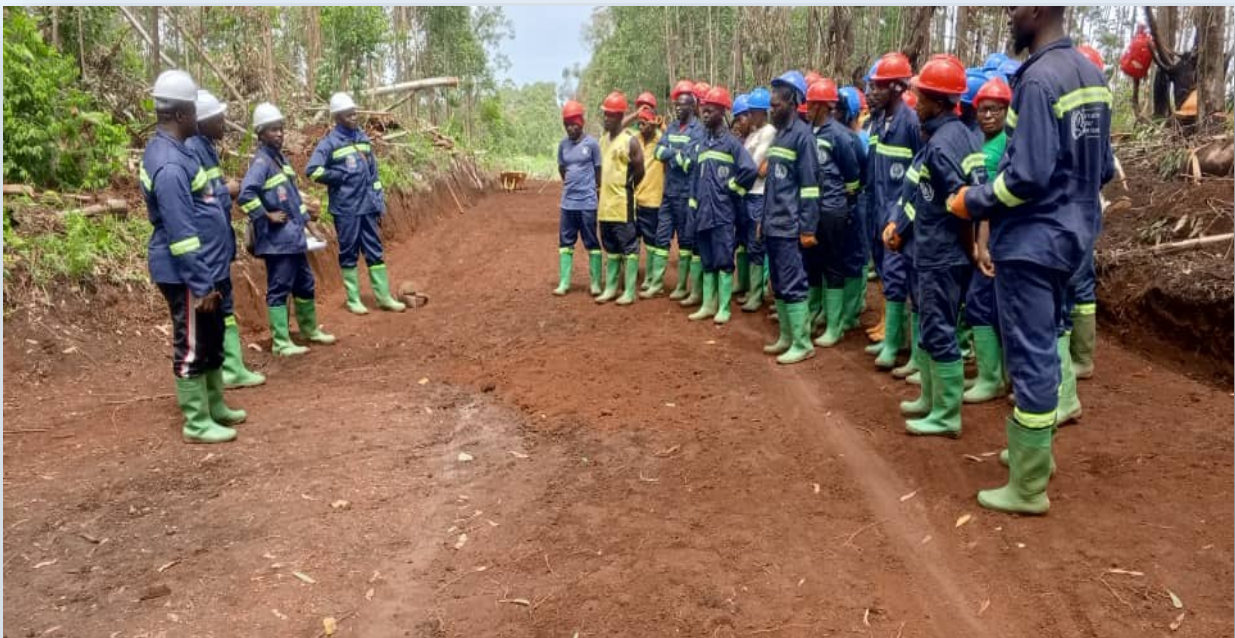
Trainees of the Ndu chantier-école receiving morning briefing dressed in their PPE before the start of work
