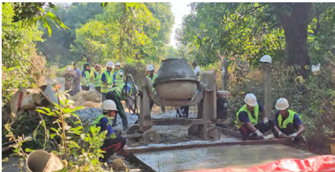
Workers working on concrete pavement
