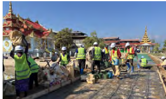
Road rehabilitation works
