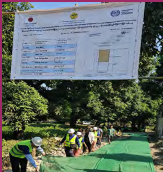
Site safety measures during the road rehabilitation works in Mandalay Region
