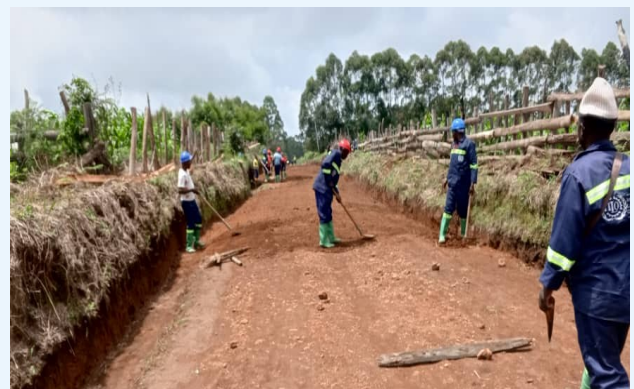
Moulding of carriageway in Ndu Council
