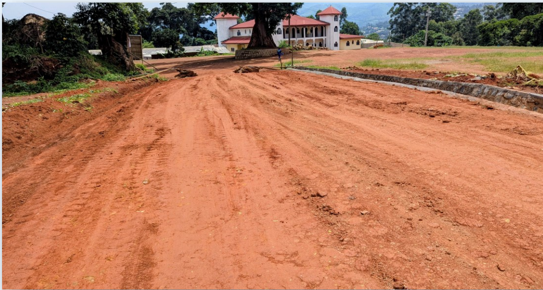
Carriage way moulded by trainees in Tubah Council and manually compacted
