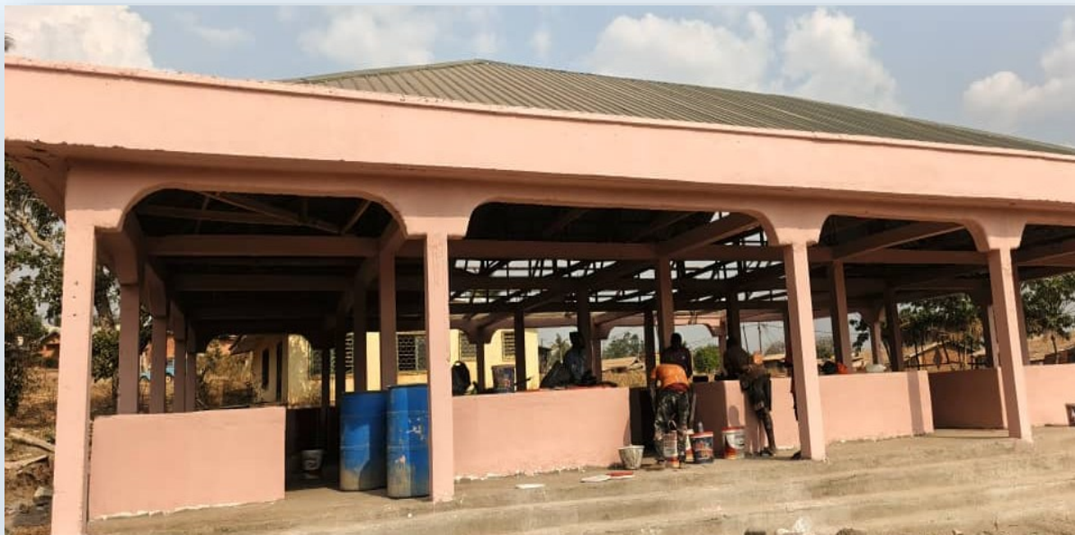
Picture of market shed in Ndop under construction
