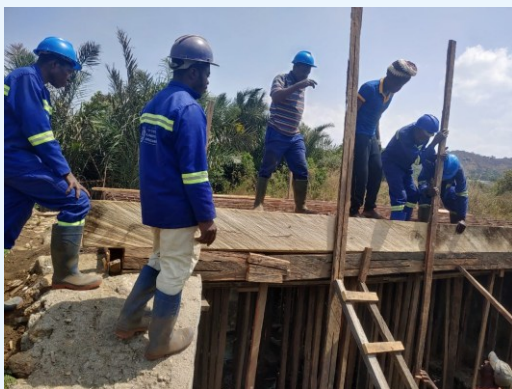
Construction of a bridge in Fonfuka Council
