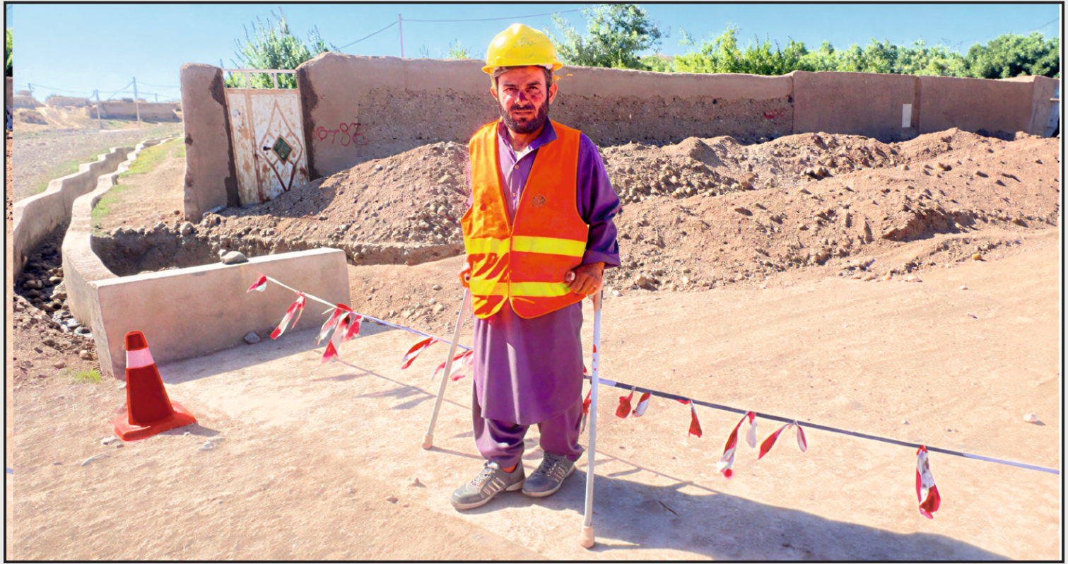
Figure 1: Nesar Ahmad Zuri works on a road project in Khwaja Qasim village
