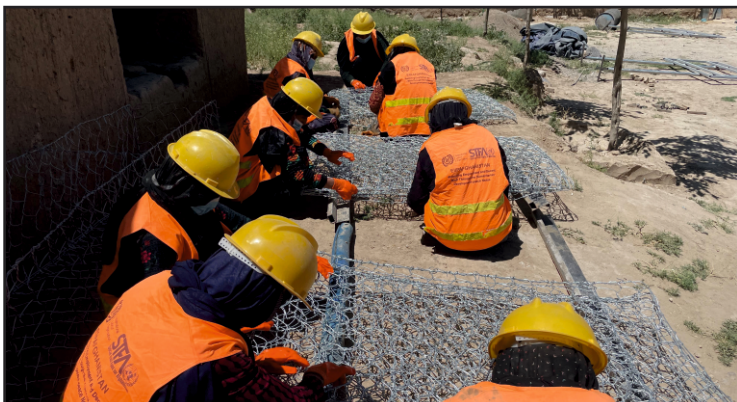
Figure 7: Gabion basket weaving activity carried out by womenworkers as part of ILO-supported infrastructure works in Kushk Robat Sangi District, Herat.
