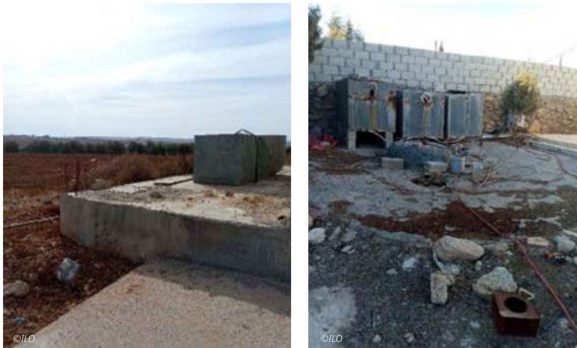
► Photo 1. Field photos: farmers using metal tanks to expand water storage capacity in addition to the water harvesting unit
