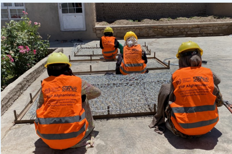
© ILO / EIIP Community Liaison Officer Women Workers weaving gabion baskets for use at construction site.
