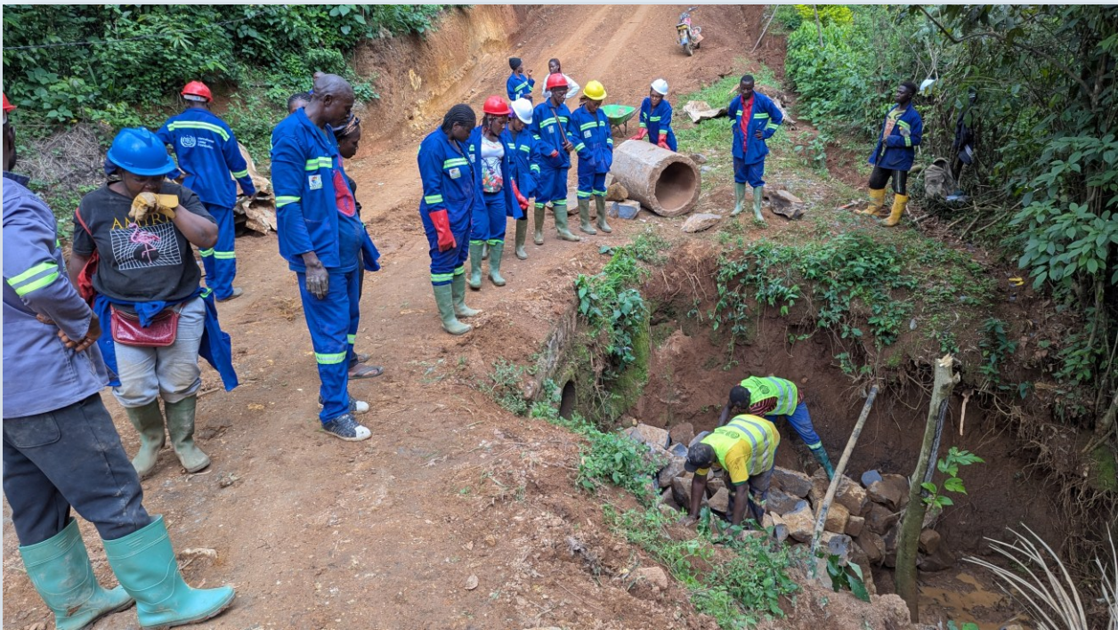
Group picture of the participants observing how to arrange a culvert using stones.
