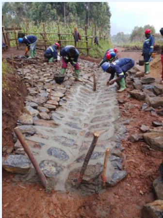
Construction of a gutter to facilitate the passage of vehicles into a church premises along the road stretch.
