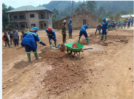
Female trainees championing the moulding of carriageway in one of the sites.
