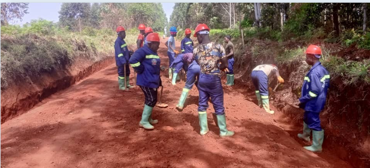
Trainees in one of the sites moulding the carriage way under the supervision of the implementing partner engineer.
