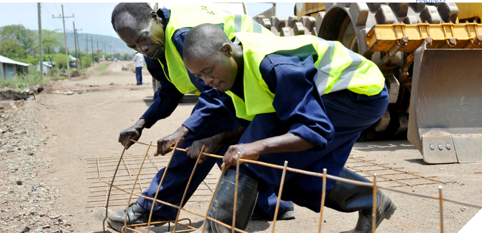
Construction workers doing road work in the streets of Suba, Kenya. © Marcel Crozet / ILO
