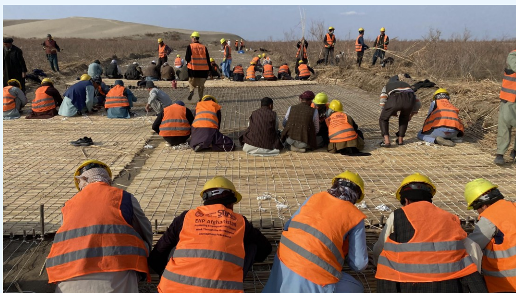
©EIIP Afghanistan: Manufacturing Bamboo Composition Layer, Shoretepa District Road Rehabilitation, Mar-2024
