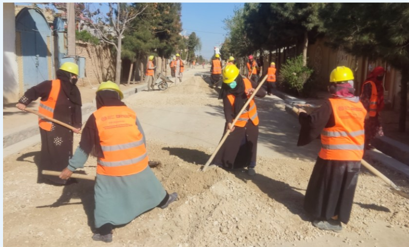
©EIIP Afghanistan: Women workers engaged in subbase spreading, rehabilitation of Khalid bin Walid Road, Mazar-e-Sharif, March 2023
