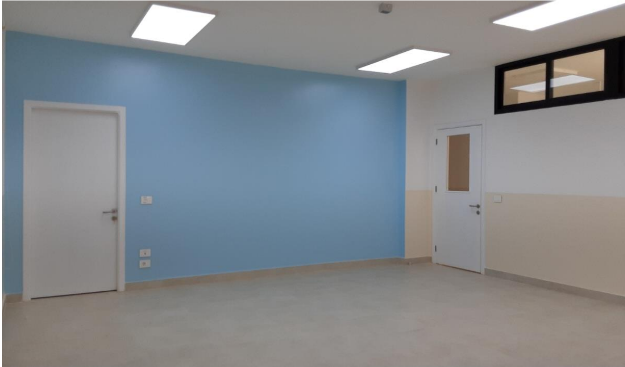
9-G.1- Internal Paint
