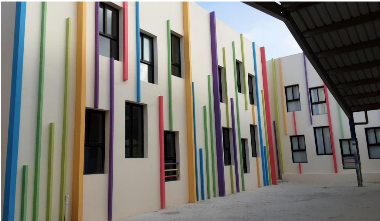
9-G.2- External Paint
