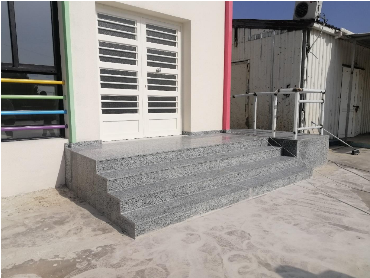
5-Metal works (supply and install hinged metal doors)
