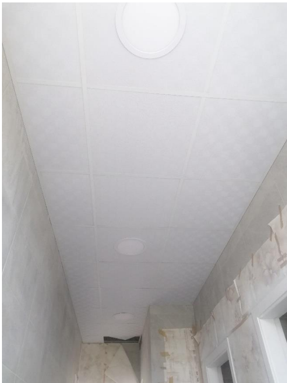
9-C-Gypsum board suspended ceiling
