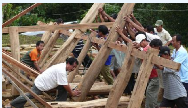
Houseowners and skilled carpenters erecting a traditional house on Nias Island, Indonesia. 05/2010, © Andreas Beusch/ILO
