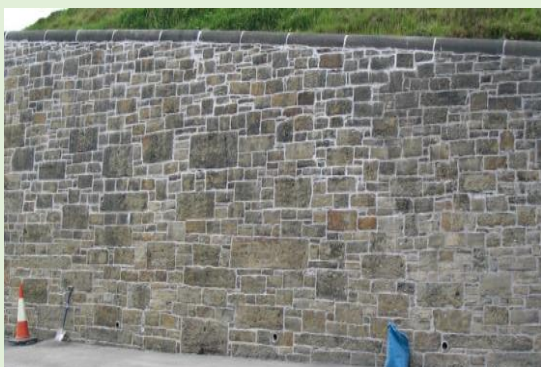
Masonry walls, cement bound or without
