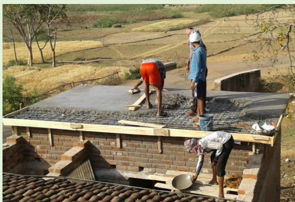
erecting shuttering and concreting slabs ...
