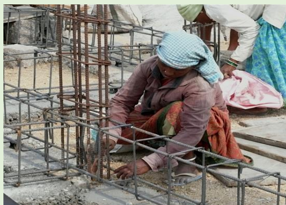
to cut, bend and tie concrete reinforcement bars ...
