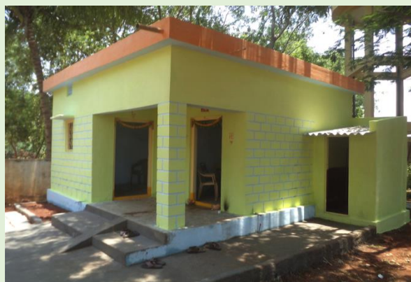
and carrying out all finishing works including plastering, flooring, painting and installing toilets with basic plumbing.
