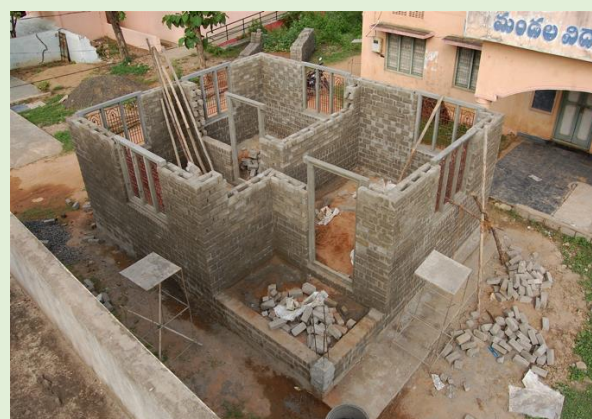
setting and installing window and door frames ....
