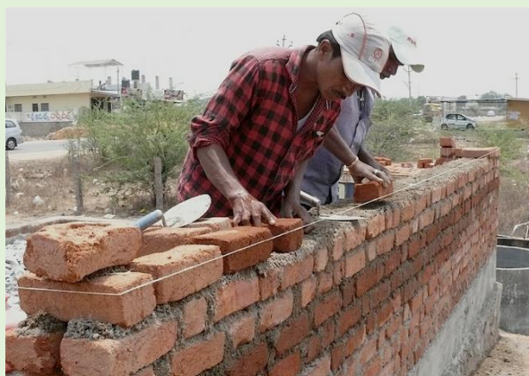
building walls using bricks or stone/cement blocks ....
