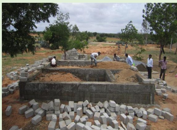
Rural masons are trained to excavate and lay foundations ....
