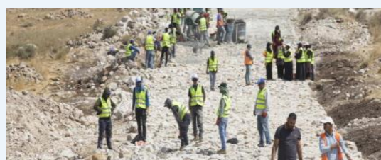
Photo 5: Stone pavement for a rural road in alKoora Municipality under EIIP Jordan Phase I
