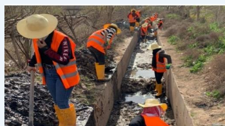
Photo 1: Repairing and cleaning 50 KM of water irrigation channels in the Kurdistan Region of Iraq
