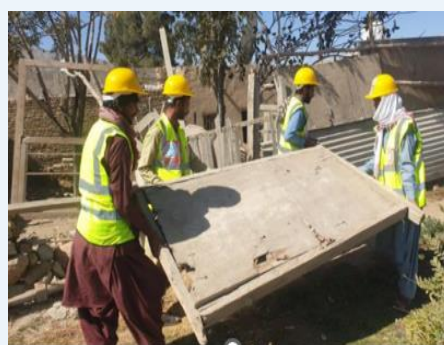
Photo 9: ILO Rapid infrastructure rehabilitation project for the flood-affected people in Hunna Orak, Pakistan
