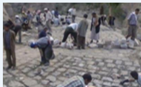
Photo 8: Social Fund for Development maintenance and pavement to rural roads to combat climate change in Yemen
