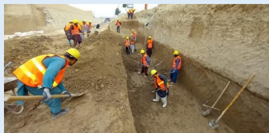
Photo 3: EIIP Afghanistan Tasadi protection wall project
