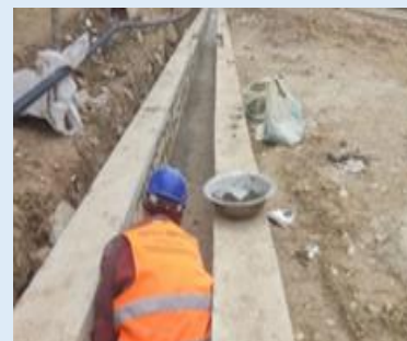
Photo 4: Khalid bin Waleed Road rehabilitation project
