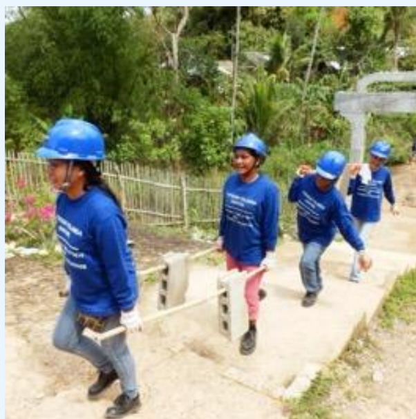
Post-Haiyan typhoon rehabilitation project, Busuanga, Palawan, Philippines, ©ILO Haiyan, 2015
