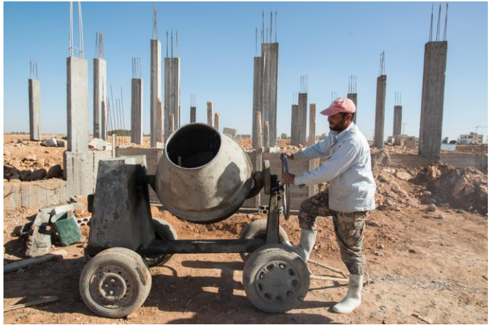
Construction worker. Jordan. 2014/12 © Nadia Bseiso/ILO
