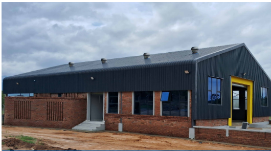
An outside view of the completed Hauna banana processing plant building. © ILO 2024, Zimbabwe
