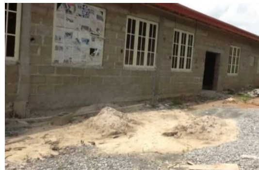
Ogun state Family Court under construction
