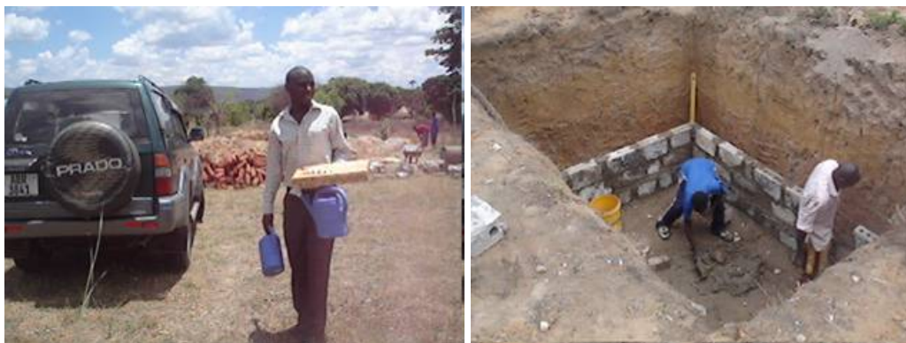
Figure 2: Community Volunteer Mr. Ngulube (left) and Builders Constructing a Toilet for the Centre
