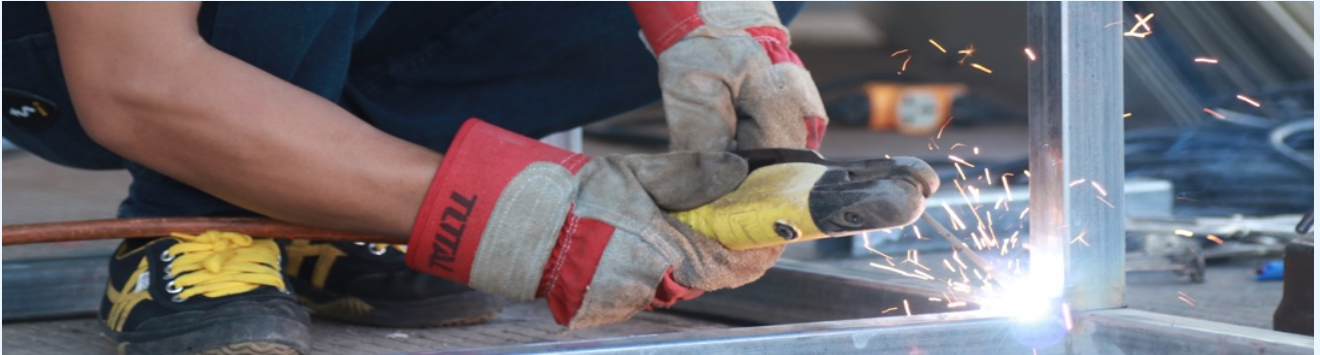
A worker uses protective gloves to protect against electric shocks while joining steel © Mongkon Duangkhiw/ILO
