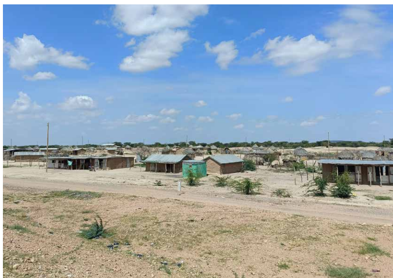
Mini-grid site in Turkana County. © ILO/Collins Oyuma
