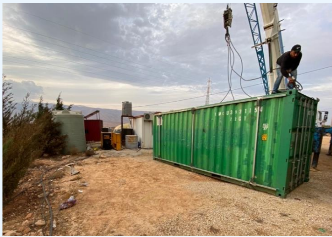
Process of installation of portable solution
