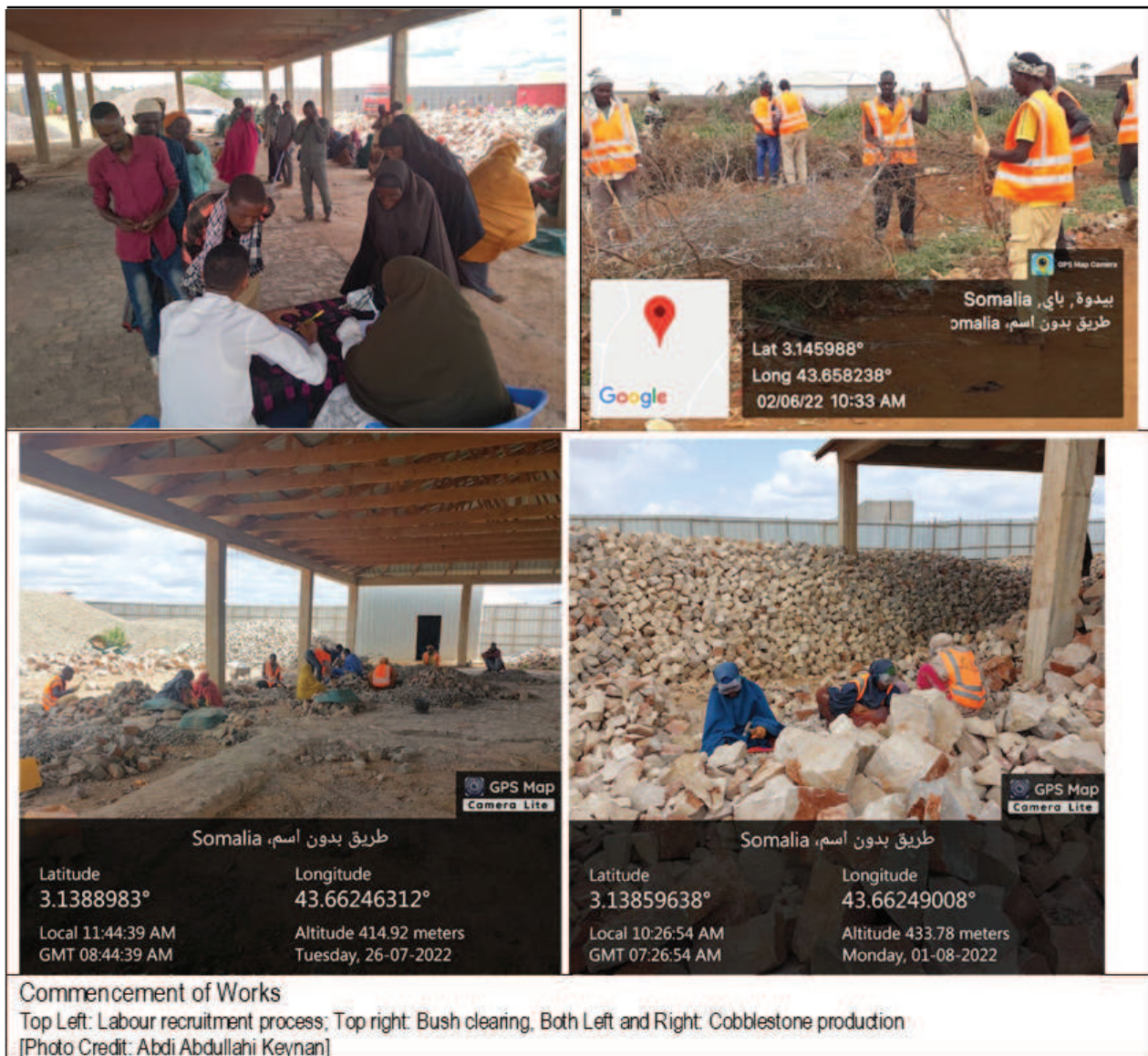
Photo 1: Commencement and preparatory works
