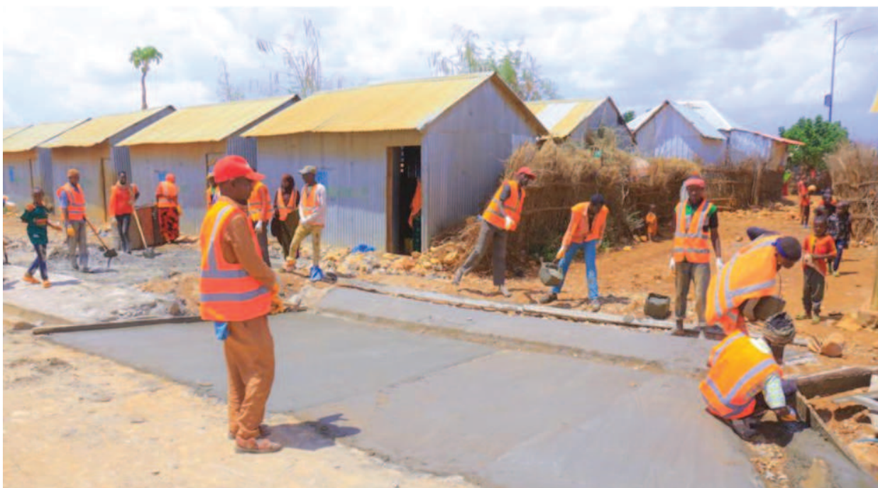
Photo 5: Construction works - cross drainage
