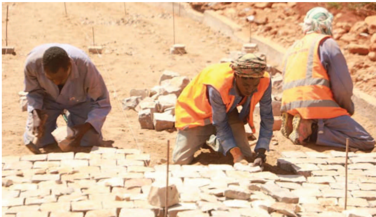
Photo 4: Construction works - cobblestone paving
