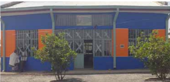
A banking branch for DECSI has been constructed and furnished
