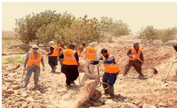
Figure 1: Rubble Cleaning activity, Zindajan District, Herat Province
