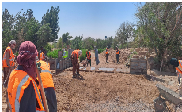
Figure 2: Road Formation Work, Zindajan District, Herat Province
