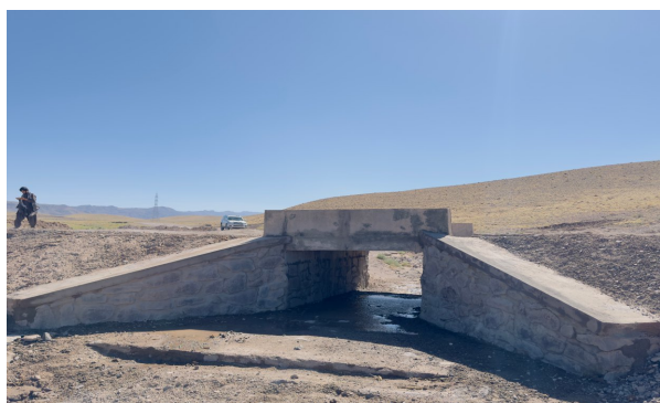
Figure 3: Culvert after construction, Zindajan District, Herat Province
