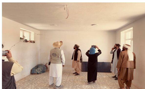
Figure 5: Assessment of earthquake damage in a school building, Earthquake Affected Areas of Kushk Robat Sangi District, Herat Province
