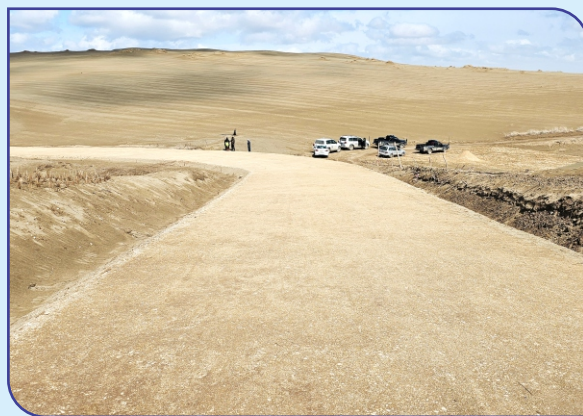
Shortepa District Road After Rehabilitation
