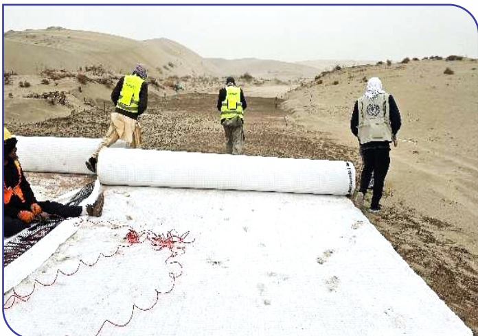
Laying Geo composite for Stabilization of Subgrade
