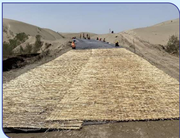
Using Bamboo Composite layer for Stabilizing Subgrade
