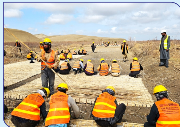
Manufacturing Bamboo composite on Project site
