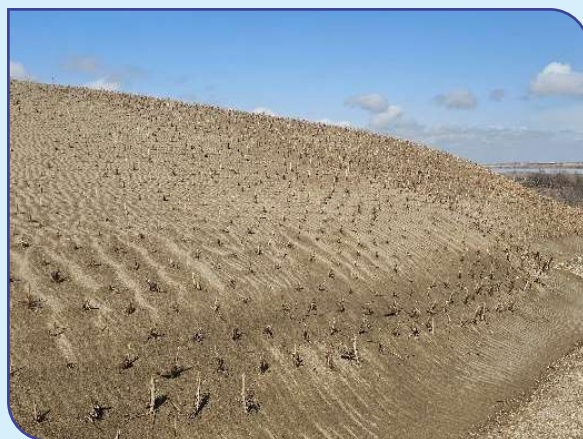
Bio Engineering, Cherkas Bushes Plant for Slope Protection
