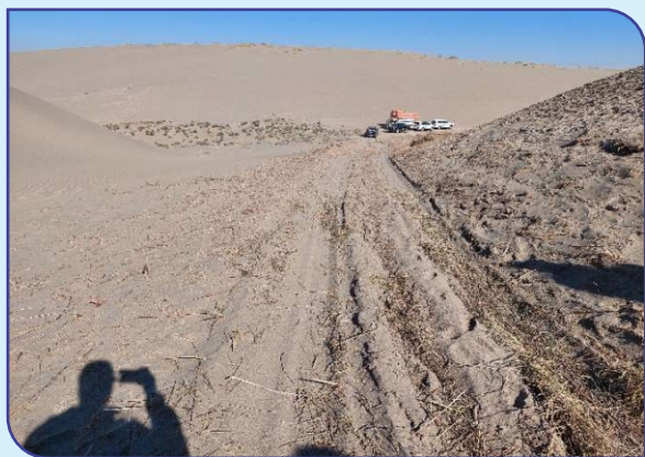
Shortepa District Road before Rehabilitation
