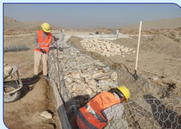
Filling Gabion Baskets
