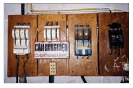
During maintenance, the control should be locked and have a tag "DANGER! DO NOT OPERATE".
