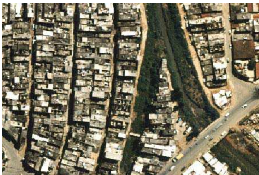
Picture 2 – Substandard housing in Osasco
