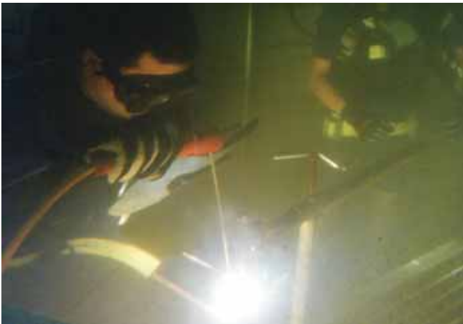
Underwater welding demonstration in Songkhla.
