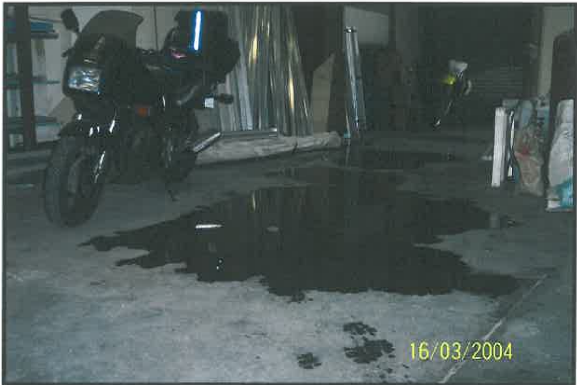
Photo 1 – Pool of Water on Floor
