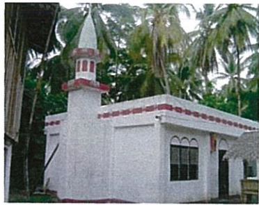
A Mosque in Mindanao. Access to water supply makes it easier for the community to perform their religious rites.
