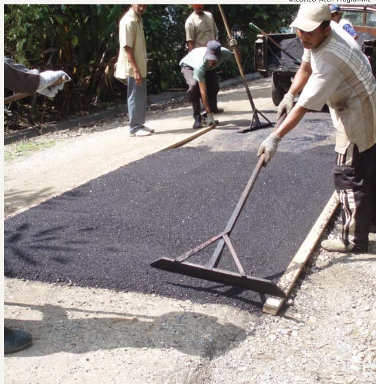
Local community built a road in one of the ILO's local resources-based rural infrastructure in Aceh.
