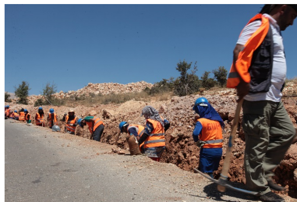
Deir el Ahmar trench excavation
