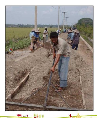
Gravel works include excavation and loading, unloading and levelling works using labour
