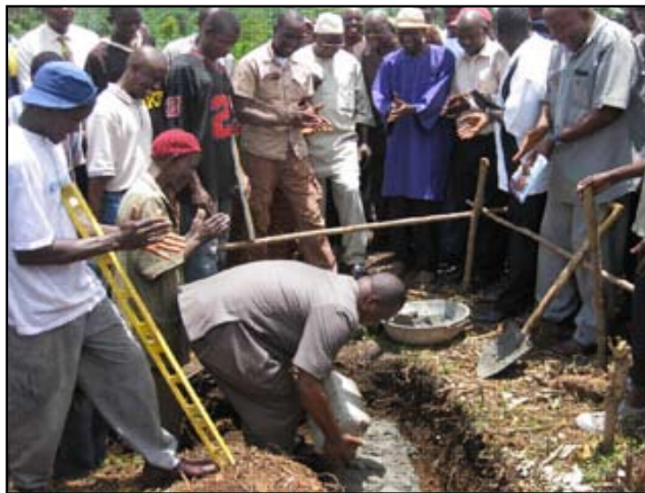
Construction du Kafoima Youth Development Centre
