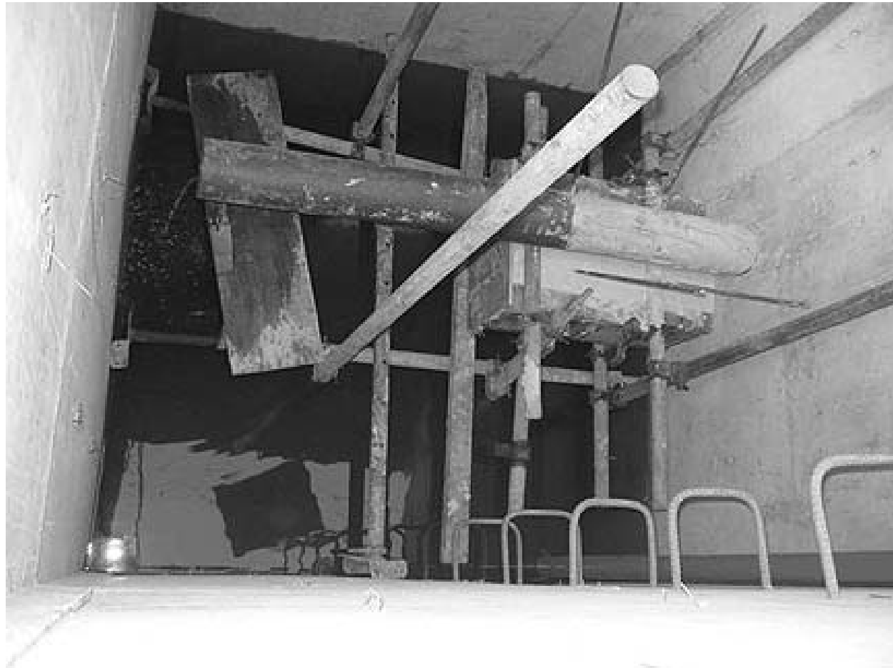
viewed from top of the pumping station chamber
