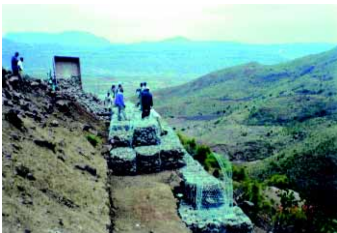
Protecting the road and surrounding environment using gabion retaining wall – Lesotho
