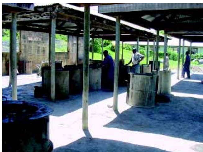
Concrete pipes production site
