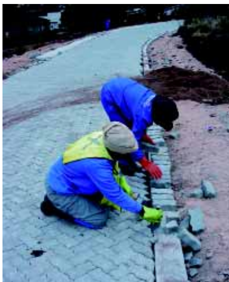
Urban road paving – a potential area of work for emerging entrepreneurs
