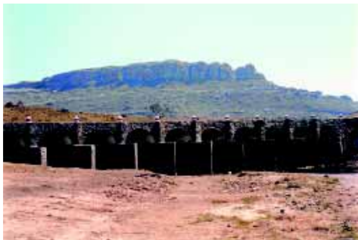
Use of local resources to improve accessibility – Masonry arch bridge – Lesotho
