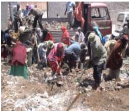
Work site in Mogadishu
