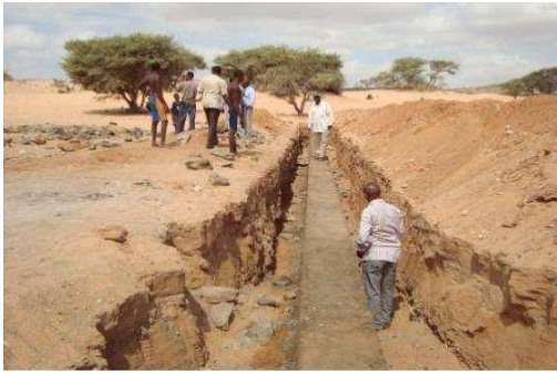
Erecting the wall across the dry river
