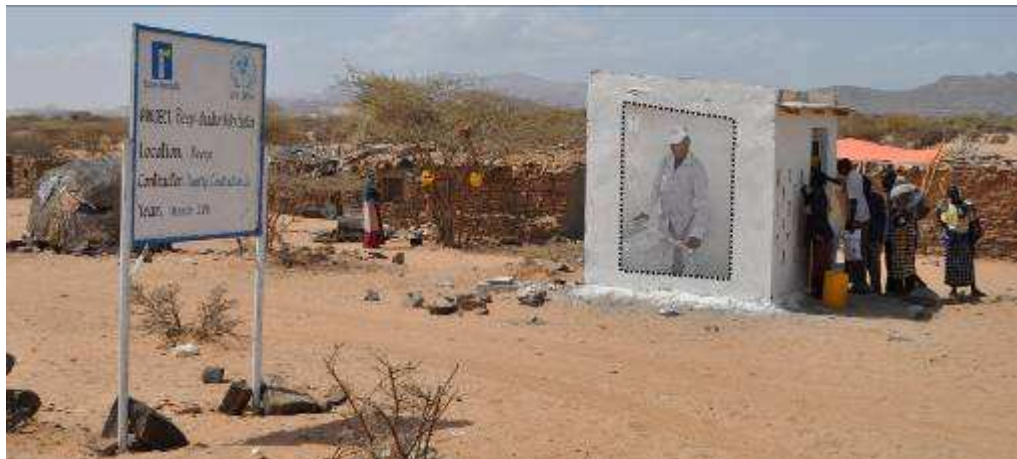
The resulting water kiosk, down the valley, that is saving the community from walking kilometres in search of water.
