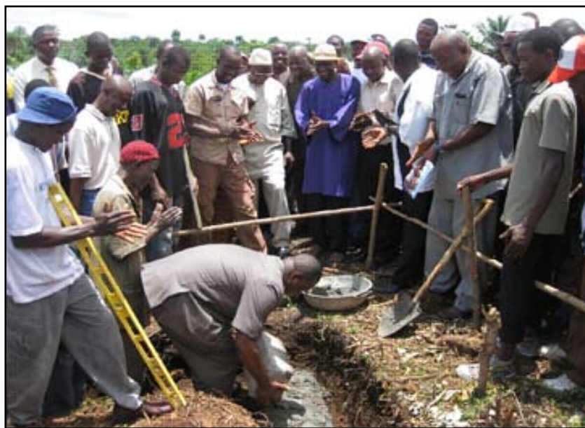
Construction of the Kafoima Youth Development Centre
