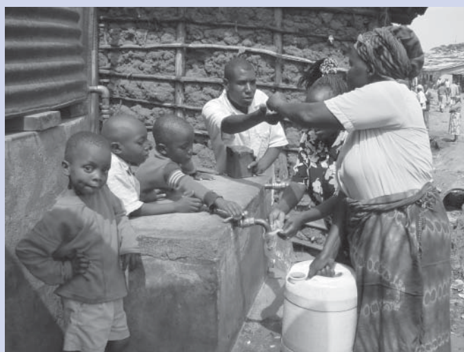
Water supply kiosk in a low income urban settlement, Kenya
