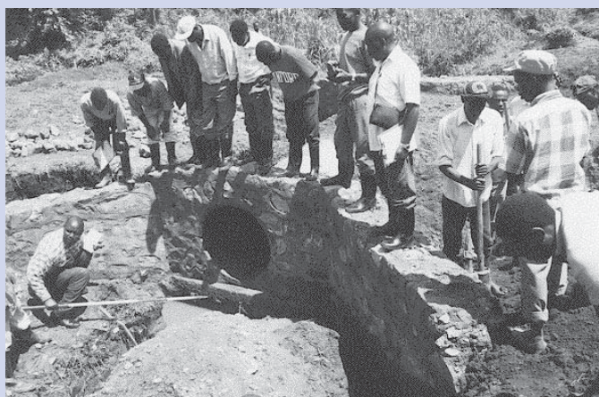
Labour-based roadworks field site training, Zambia
