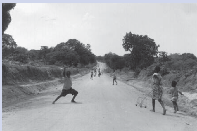
A complete gravel road, Mozambique
