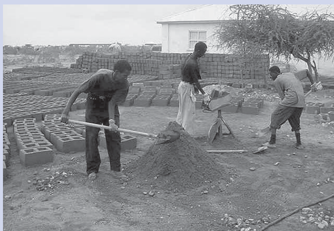
Block-making for low cost housing, Somalia
