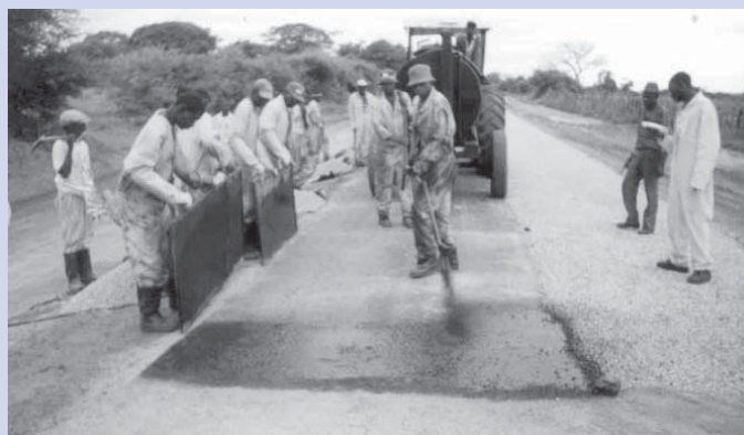
Low volume road sealing, Zimbabwe
