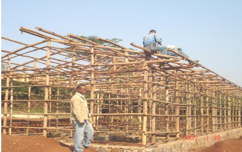
Residential houses for teachers under construction by the management
