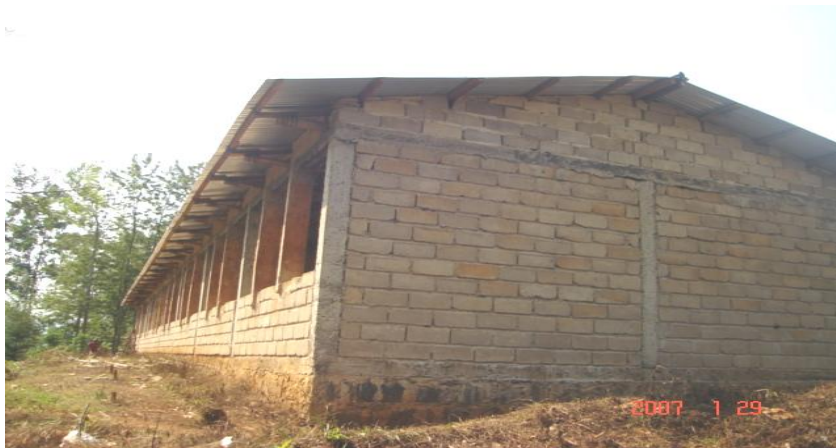
The school under construction by the management
